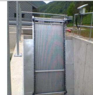
Siapro provides all hydro machinery equipment, for example coarse and fine grids in various configuration. Coarse grid is installed at the beginning of hydro power plant intake facility to remove impurities: stones, wood, etc..
